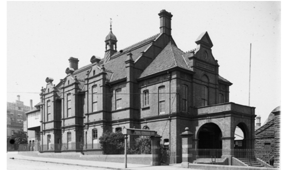
Railway Institute Building 1919 (Source: NSW State Archives)
