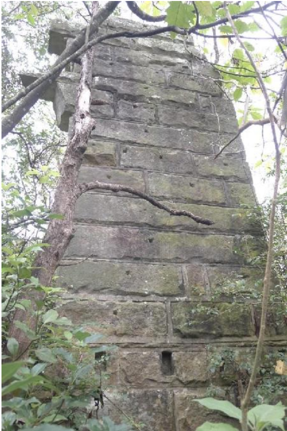
Figure 4.12 Detailed view of the sandstone wall relating to the Powderworks, believed to be part of the original Office and Magazine building. Checkouts are visible for possible timber joists and indentions indicate the position of a strucutre that was previously fixed to the wall. (Source: GML 2014)
