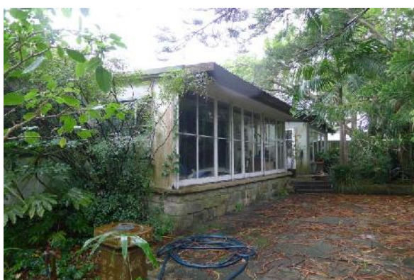
Figure 4.34 Pickerill's cottage, located in the southwest corner of the site. (Source: GML 2014)
