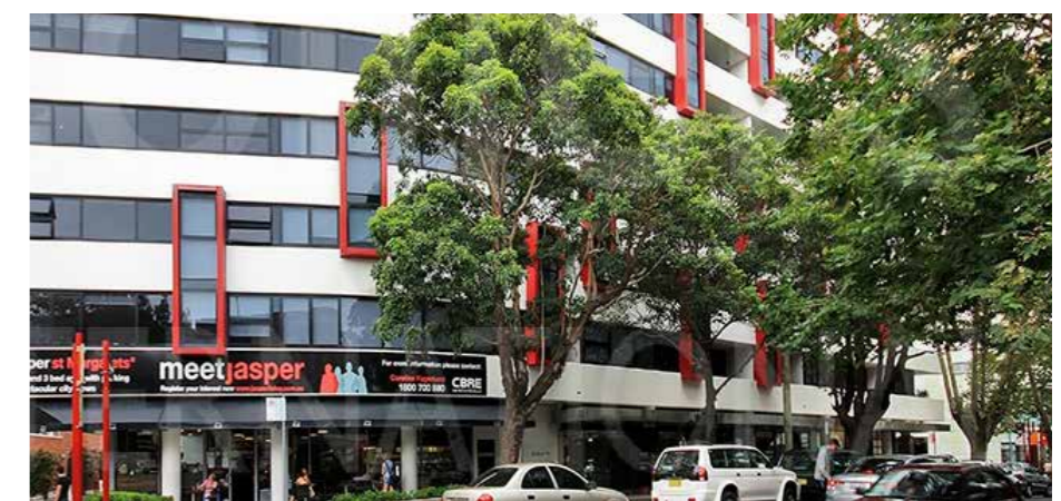
Figure 25: Proposed location of mixed use retail and residential, and desired character and built form
