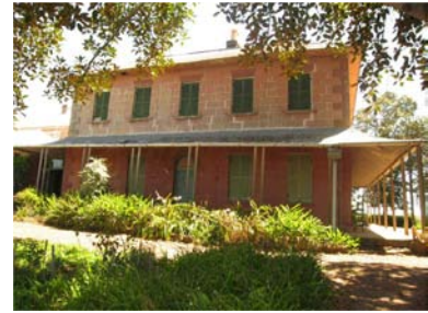
Figure 5.51 View of the south-facing elevation of Rouse Hill House, which is located within the study area. (Source: GML 2009)
