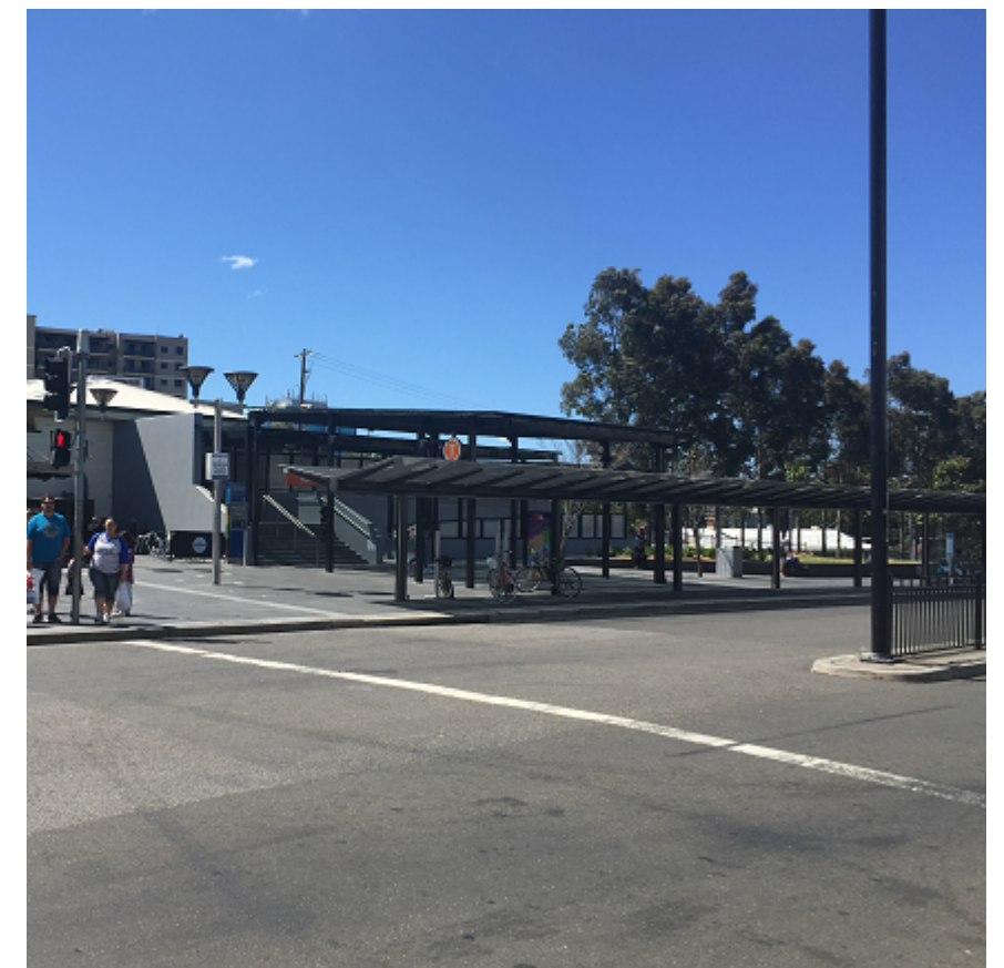
Intrusive Bus Interchange decreases overall public amenity of station precinct
