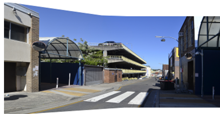
before - view down Stewart Lane towards council owned carpark including covered arcades
