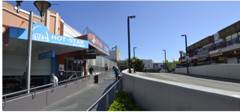
before - view towards station entry
