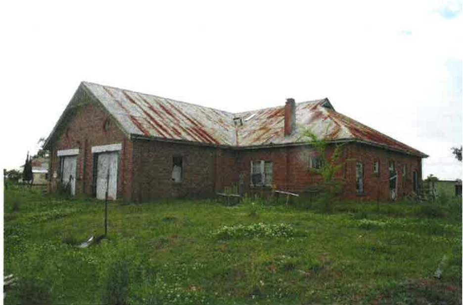
Figure 4.18 View of Clydesdale barn looking south-east
