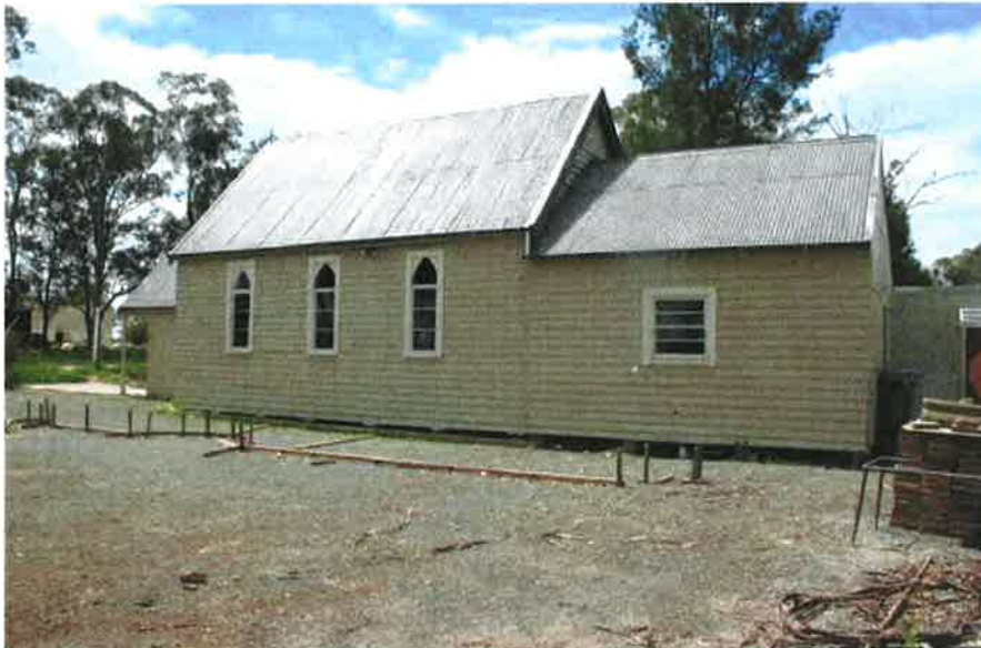
Figure 4.38 Hall, Grange Avenue
