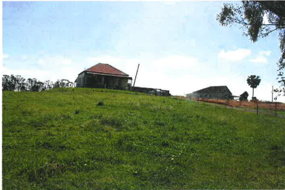
Figure 4.30 North facing photograph of Cottage at 1082 Richmond Road.
