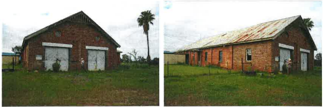
Figure 4.19 View of Clydesdale barn looking south (left) and looking south-west (right)
