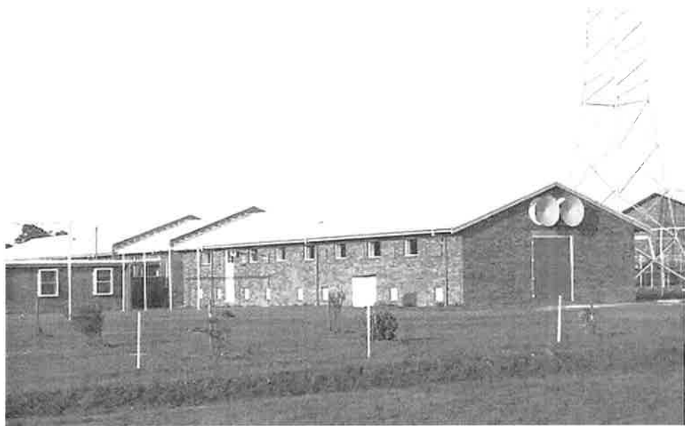
Figure 3.8 Photo from 1963 showing HF Transmitter Station (CAHS Collection).
