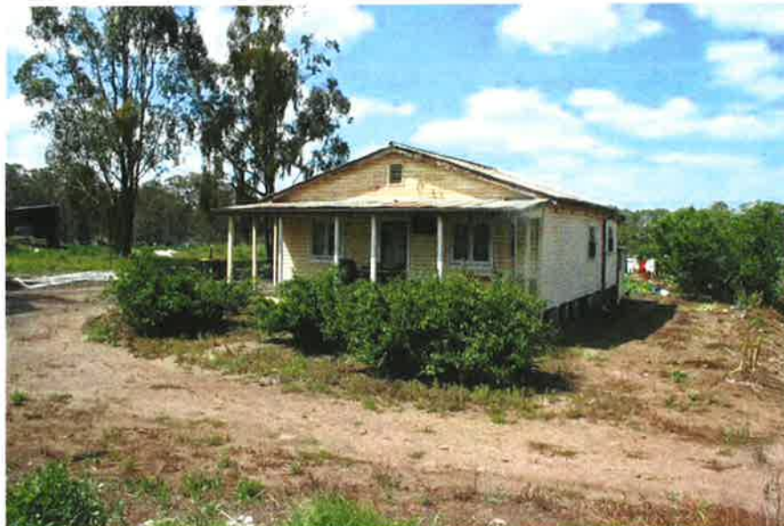
Figure 4.33 View of 1069 Richmond Road looking east
