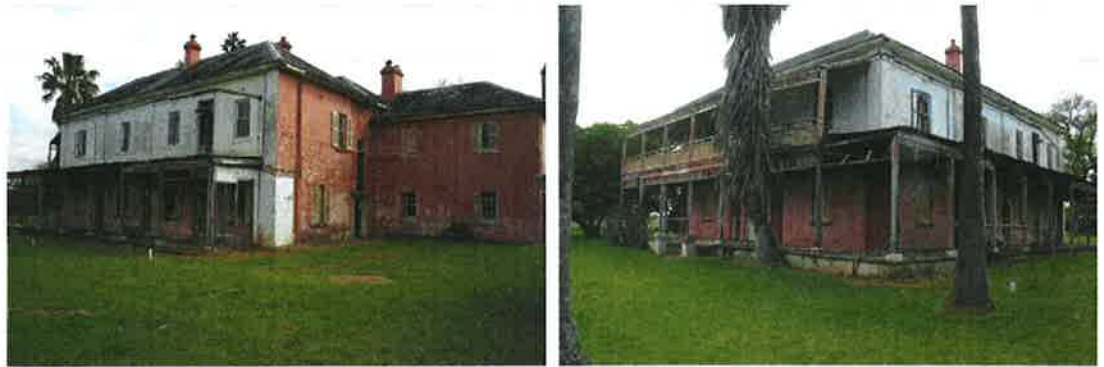
Figure 4.2 View of Clydesdale house looking north (left) and view of south east elevations with original palm trees in the forefront (right)
