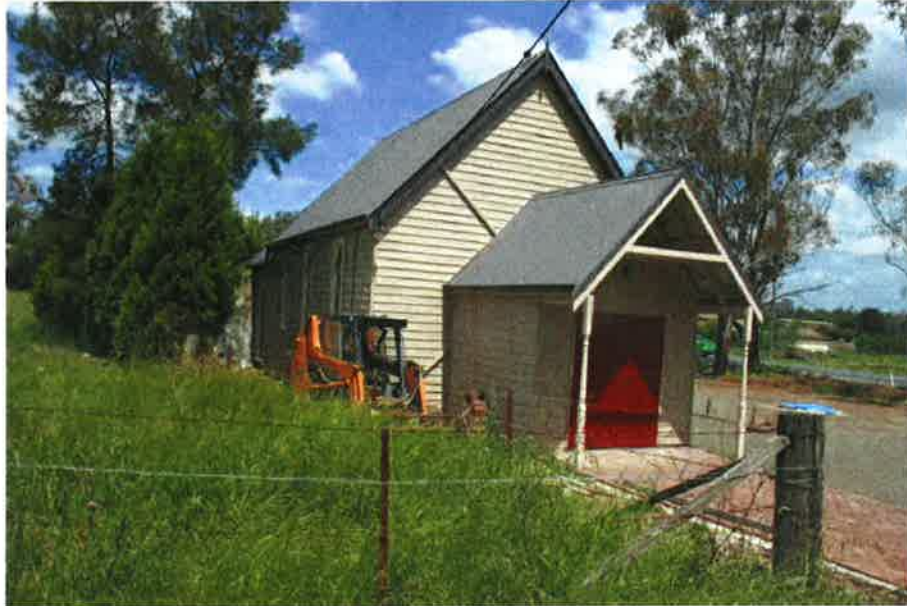
Figure 4.39 Hall, Grange Avenue
