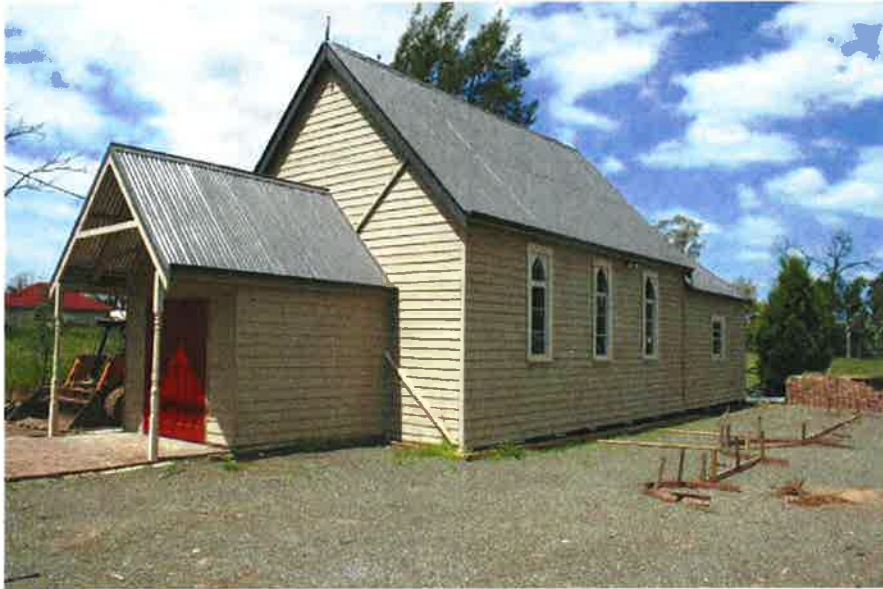
Figure 4.37 Hall, Grange Avenue
