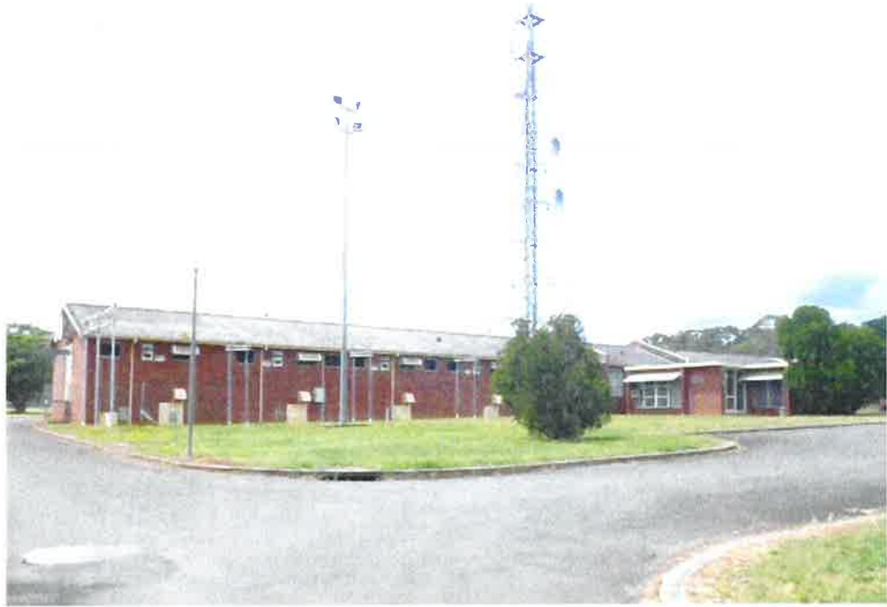
Figure 4.22 East facing photograph of brick buildings within Llandilo including antenna.
