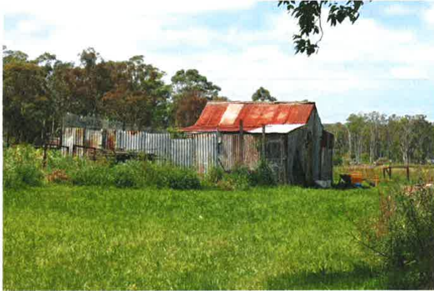
Figure 4.34 Slab cottage between Grange and Richmond
