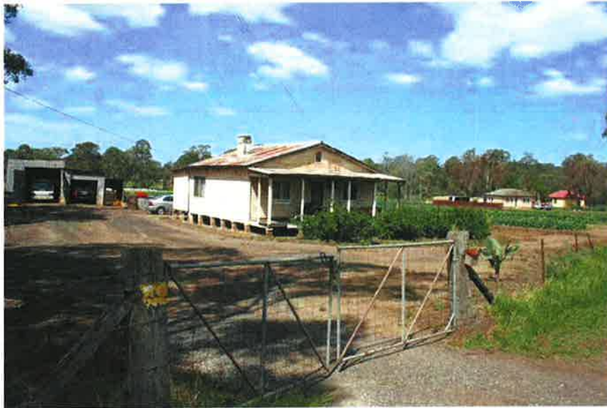
Figure 4.32 View of 1069 Richmond Road looking south-east
