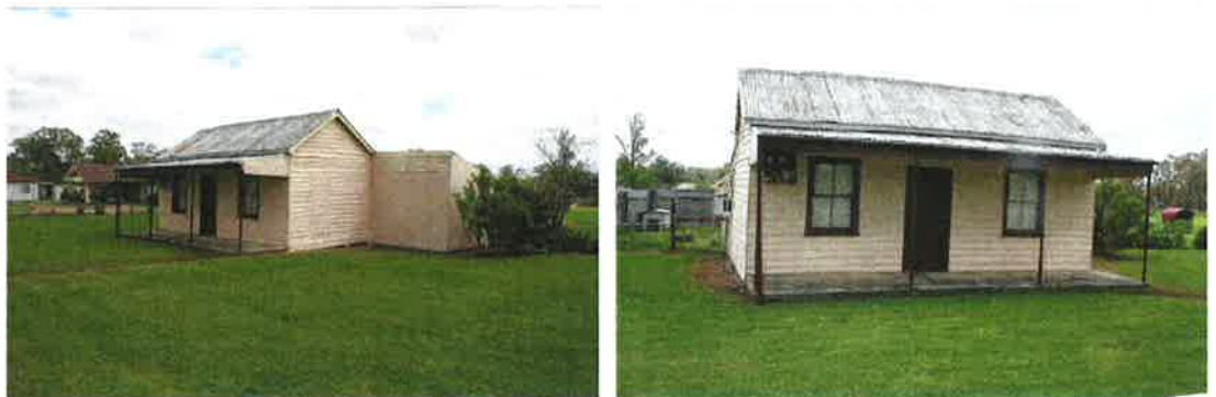
Figure 4.28 Vine Street West looking north-west (left) and north (right)
