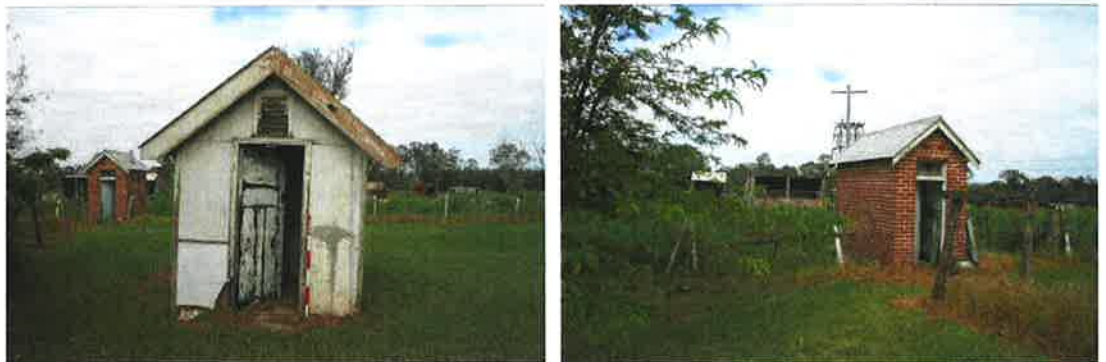
Figure 4.20 View of two privies located south of Clydesdale house(left) and detail of shed in the background of photo on the left (right)
