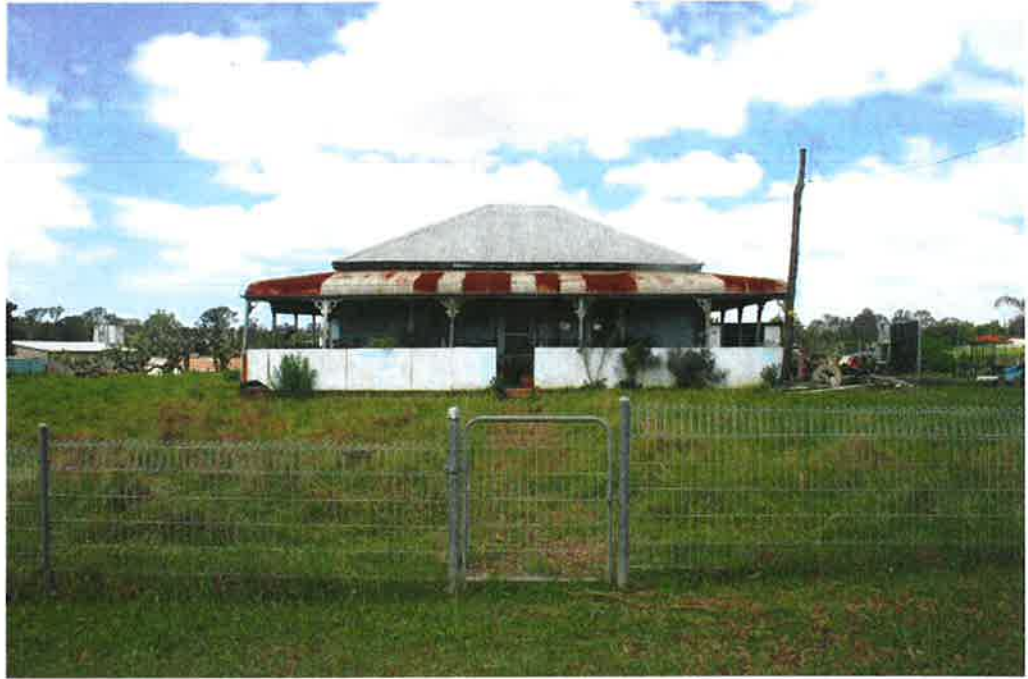
Figure 4.25 View of front facade of 142 Clifton Road looking south
