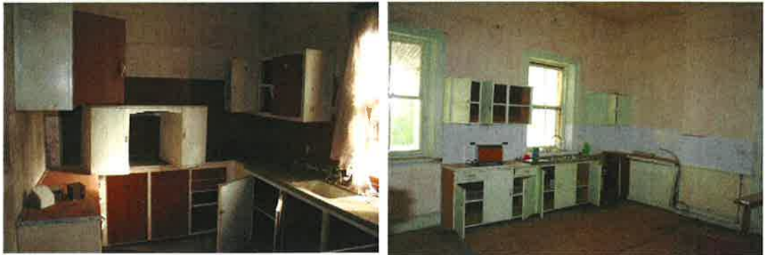
Figure 4.4 View of downstairs kitchen (left) and view of upstairs kitchen (right)
