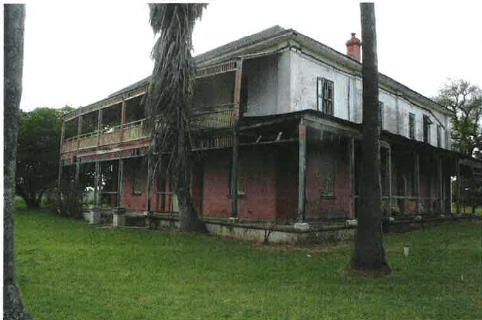
Figure 3.4 North East facing photograph of Clydesdale House c1980's
