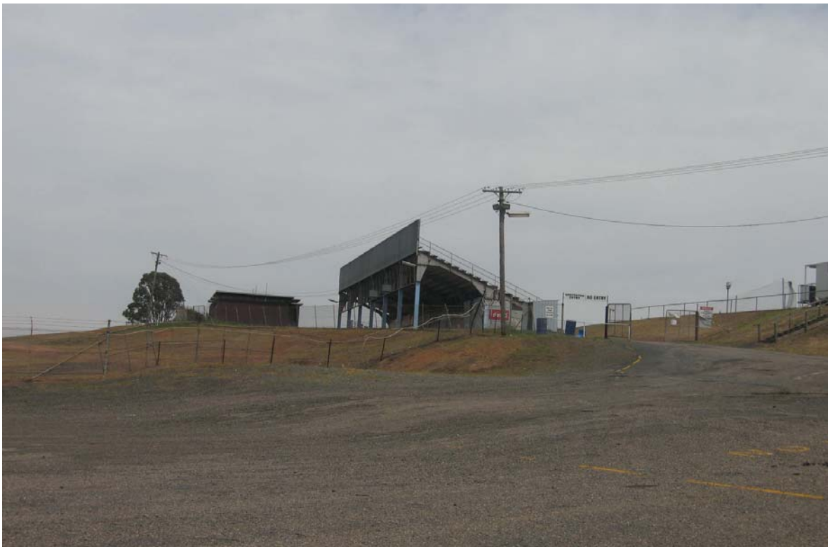
Figure 6.1 Photograph showing the main stand at Oran Park Raceway.
