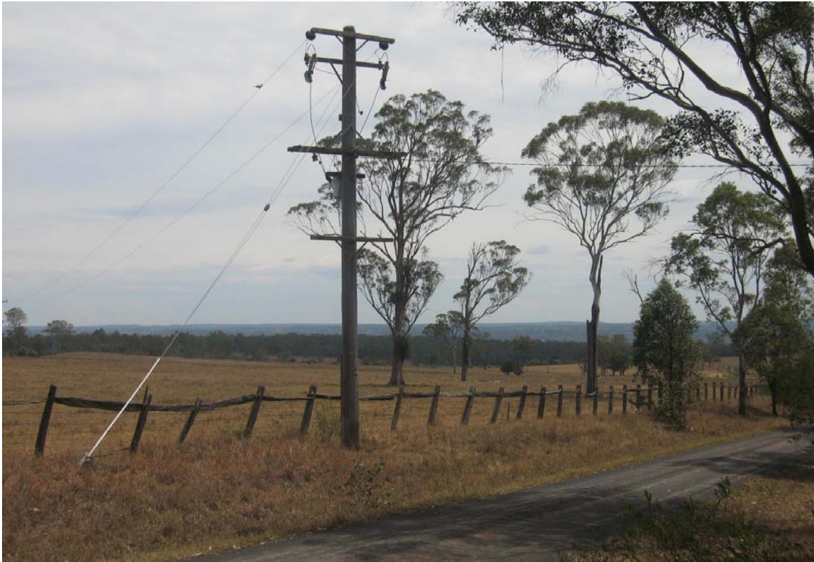
Figure 5.9 View looking southwest towards Cobbitty taken from the original entrance drive leading to Denbigh. Note the remnant fence line.
