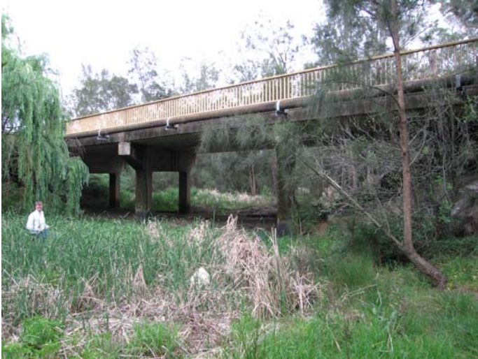
Plate 5 - Bringelly Road Bridge Looking d/s
