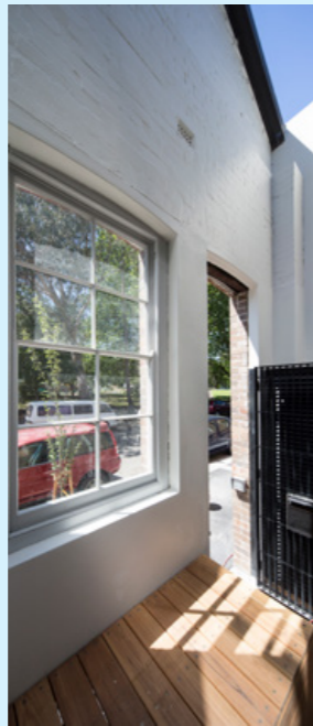
Living heritage Terrace apartments behind the retained Australia Street brick facade. Images: Brett Boardman Photography.
