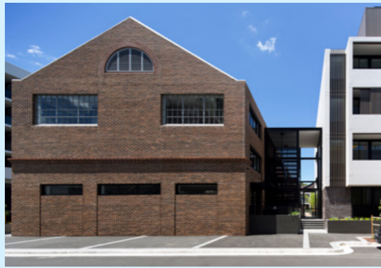
High Bay Workshop From Denison Street, the original brick warehouse is separated from the new structures on either side by an entry link and laneway. Image: Brett Boardman Photography.
