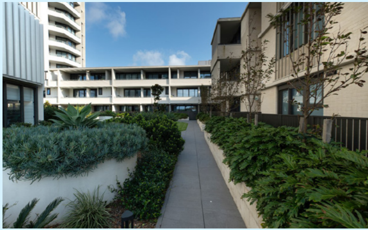
Green roof The courtyard is heavily landscaped to form a verdant outlook for residents, and includes shared facilities like edible gardens. Image: Murray McKean.
