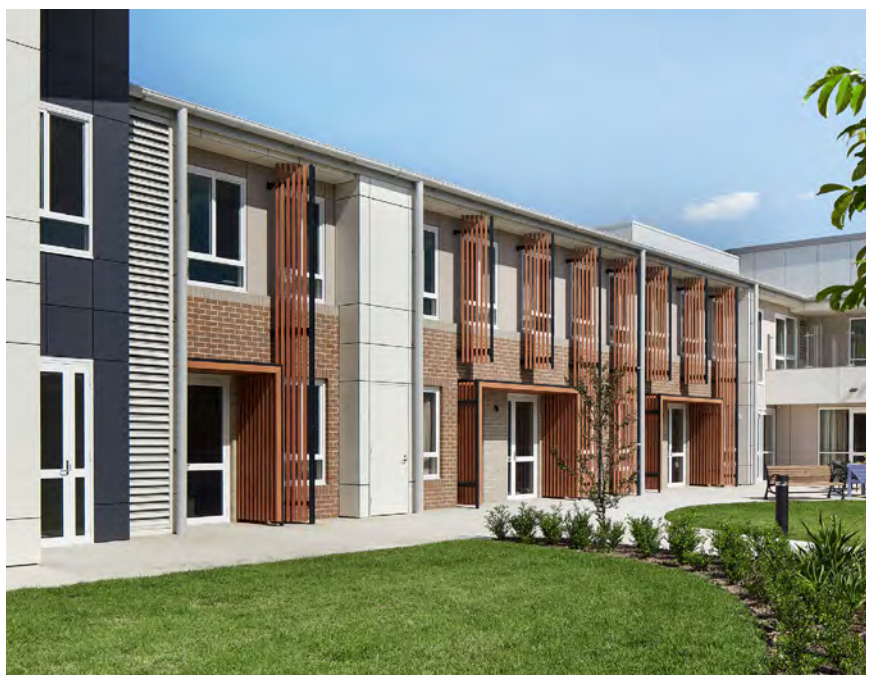
Fig 12.6.B Use screening to shade windows and articulate the façade
