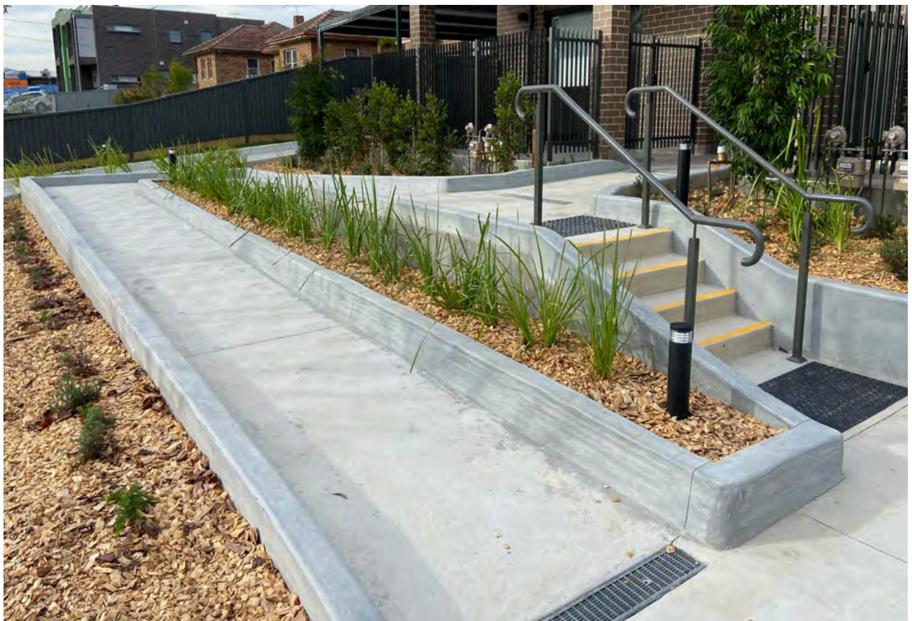
Fig 15.5.A Accessible pedestrian access
