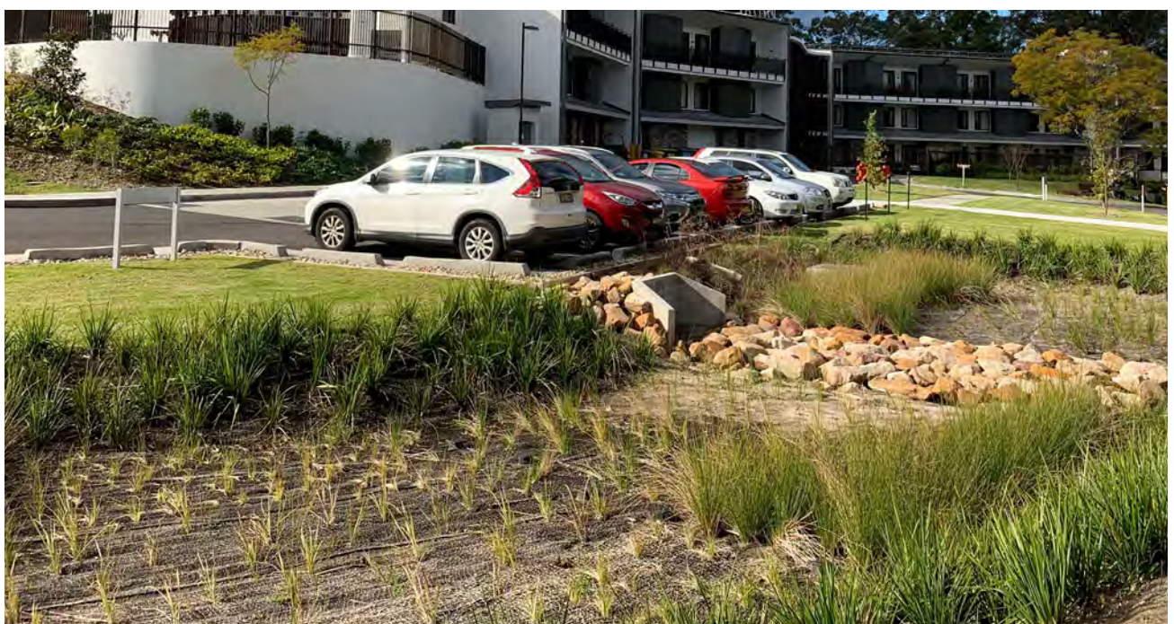
Fig 12.9.A Sensitively landscaped stormwater detention in the gardens of a residential care facility
