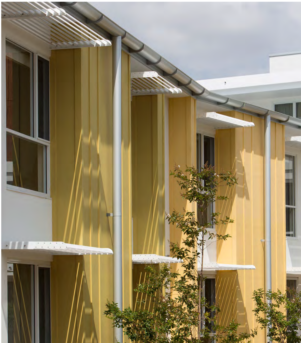
Fig 12.8.B Shading and deeply recessed fenestration articulate the external façade and provide interest with dynamic movement of shadow patterns through the day
