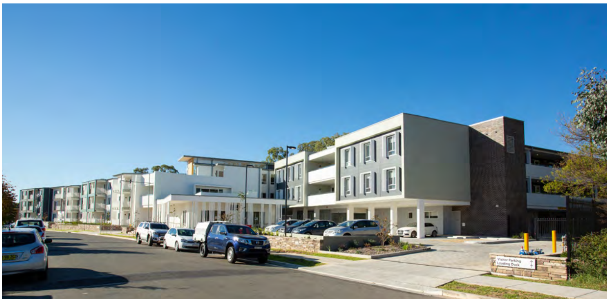
Fig 10.0.A Co-located residential care and independent living with a community centre with a range of different heights and building forms
