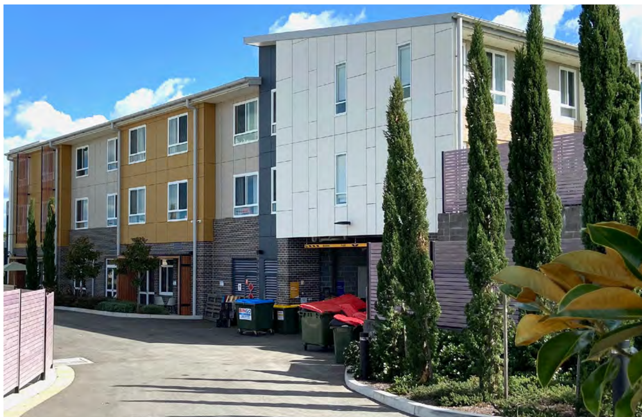
Fig 12.11.A Service driveway showing loading dock area and back-of-house utilities
