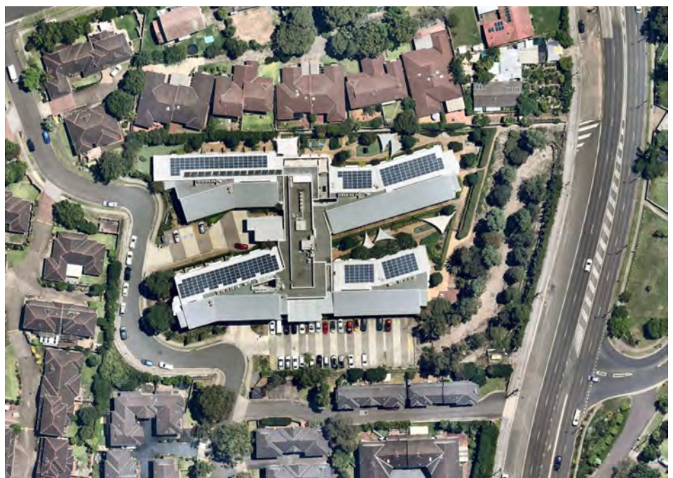
Fig 3.2.D Aerial view of completed development showing dry creek bed to channel stormwater into culvert located under carpark
