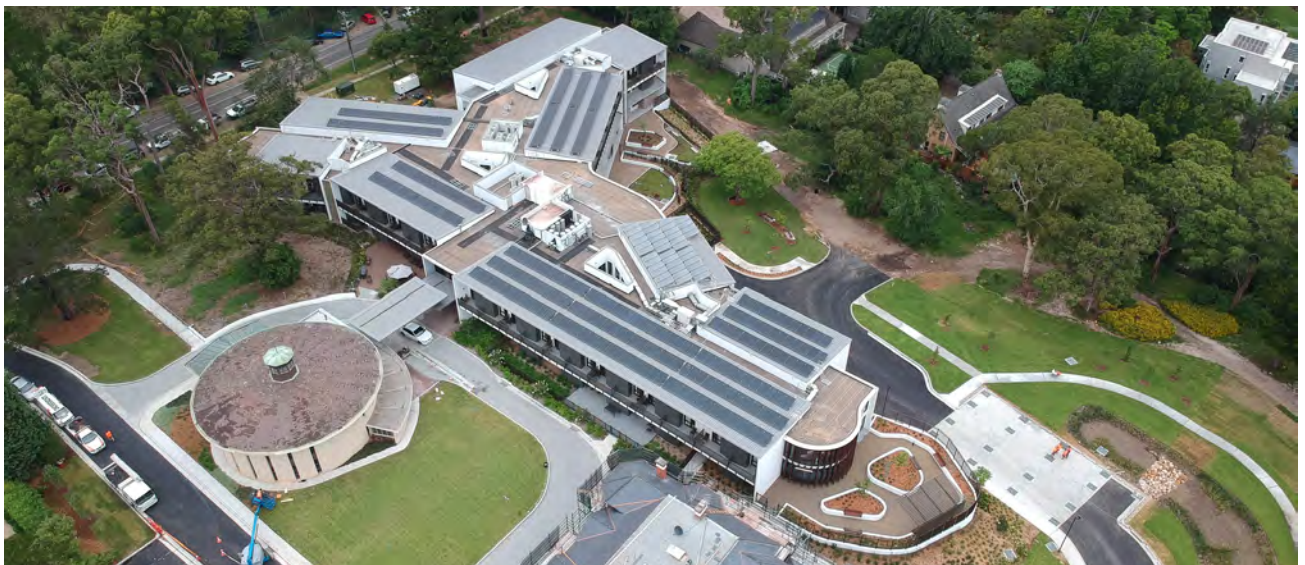
Fig 2.4.A Stand alone residential care facility with extensive photovoltaics on the roof and shading to the building envelope
