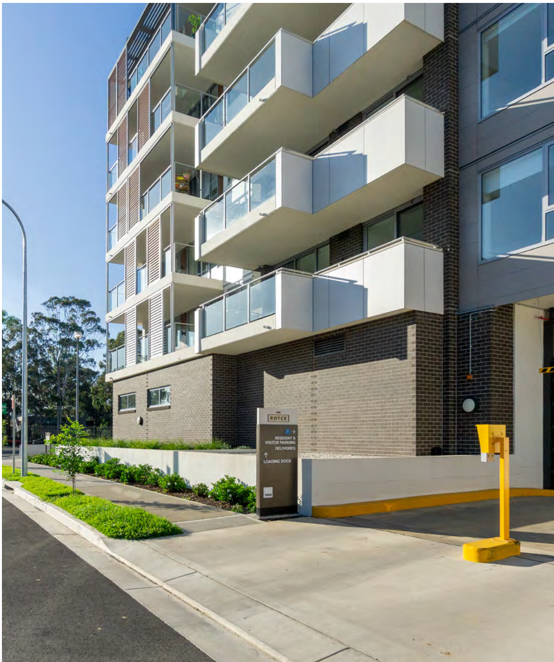
Fig 16.8.C Basement carpark entry with clear signage and level threshold
