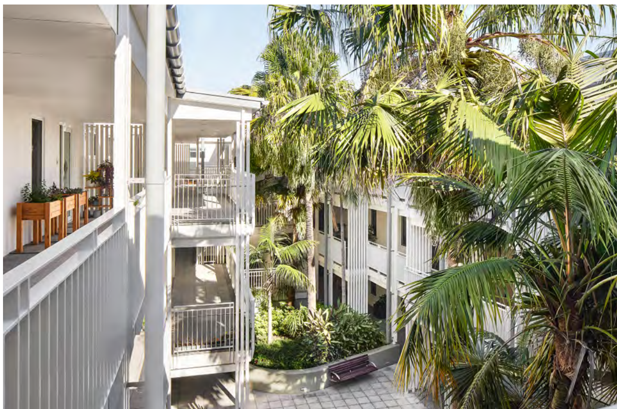
Fig 15.2.B Independent living units showing benefits of a courtyard design with single loaded walkway
