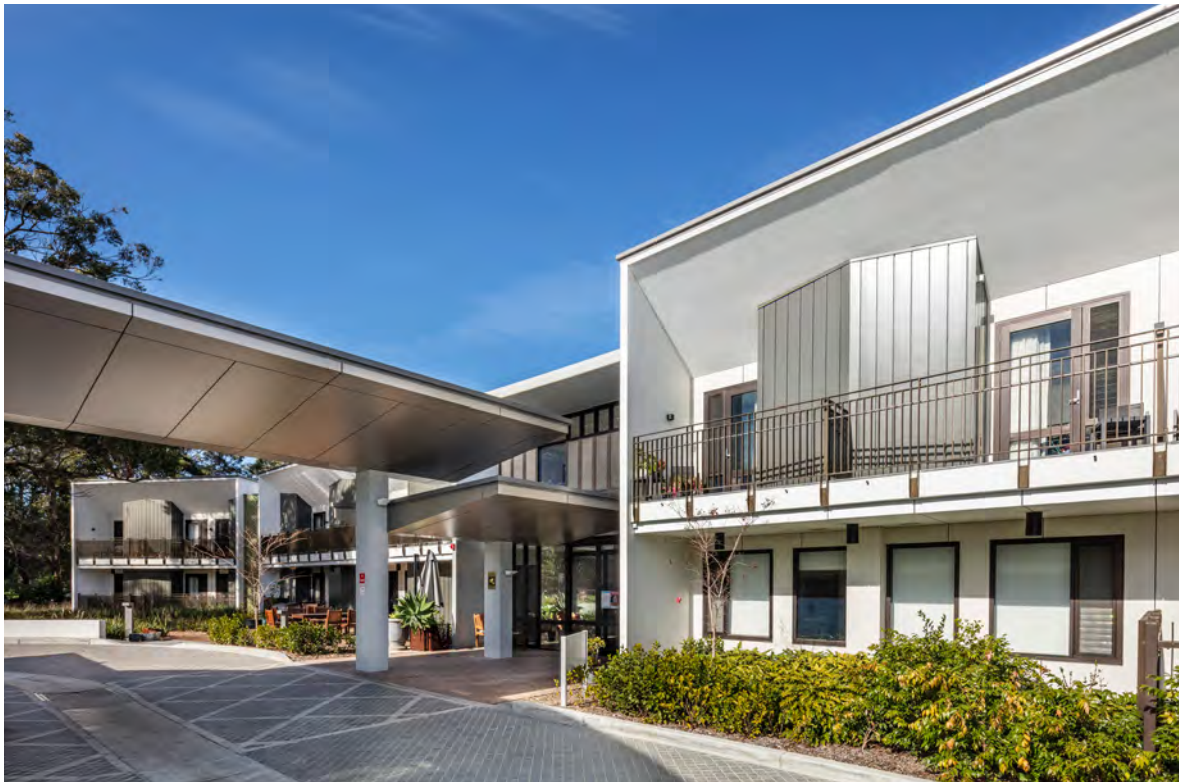
Fig 12.4.B Entry point is identifiable with generous and well-protected roof cover
