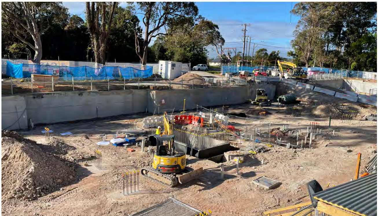
Fig 2.2.A Commencement of construction for a new residential care facility
