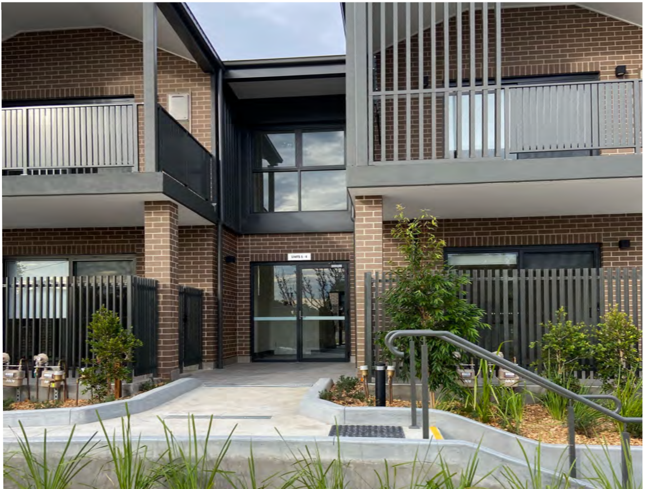
Fig 15.4.A Clearly identifiable accessible entry to shared lobby is visible from the street. Glazed doors provide visual access to the outside
