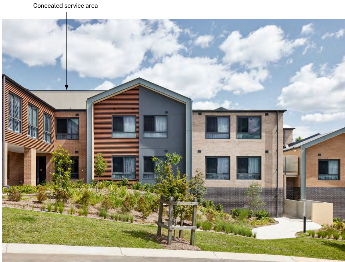
Fig 12.3.H Service plant concealed from view by roof structure
