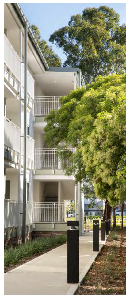
Fig 16.4.B Outdoor walkway with good lighting and sightlines
