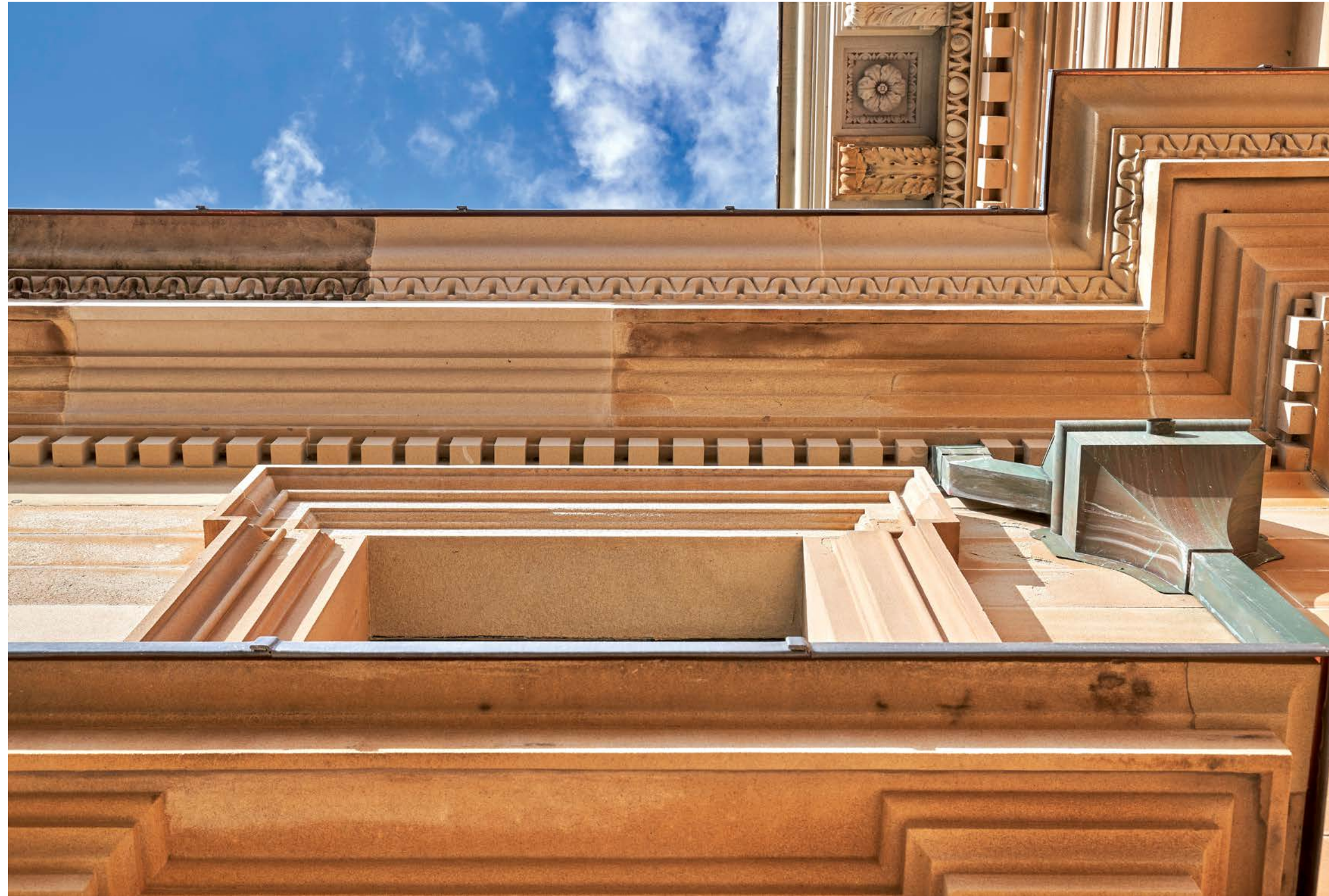
Right: The Australian Museum following façade repairs in 2020. The stone has been carefully cleaned, the open joints repointed, highly deteriorated stone has been replaced and lead weatherings have been installed to encourage water to drain freely away from the façade. Photography by Michael Nicholson, 2020.
