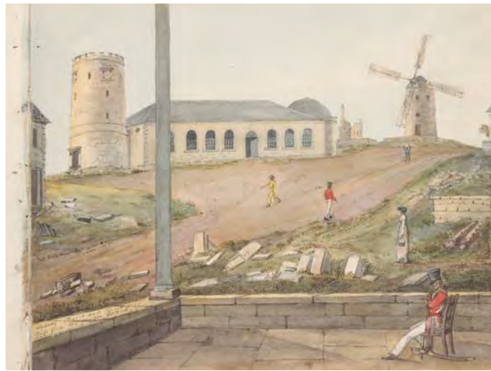
Governor Macquarie's ambitious program of public works relied on the ready availability of local sandstone. To this end he established a government quarry on the northern side of Fort Phillip (Flagstaff, later Observatory Hill) and worked by convict labour. (Detail from Sydney Church and Regimental Mill from the Main Guard by Edward Close [circa 1817] showing stone quarrying. State Library of NSW)
