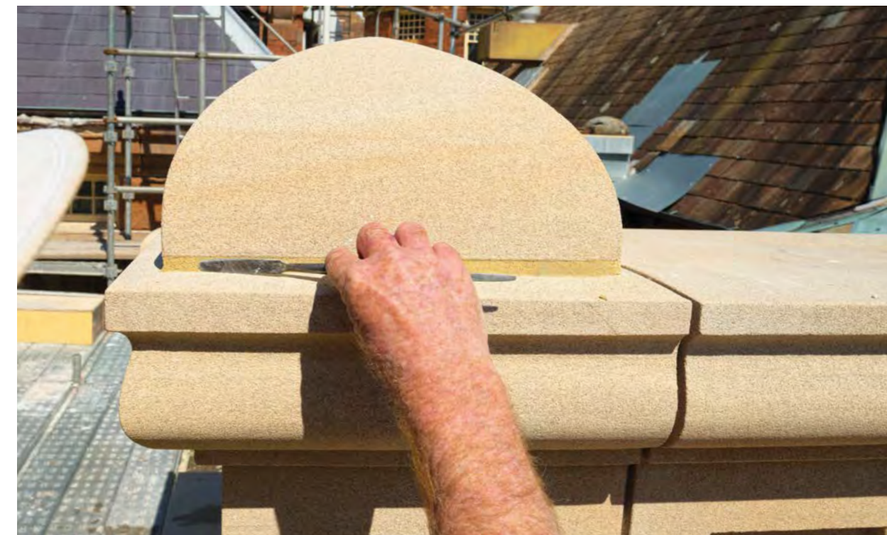
Left: Expert stone carver Luke McDermott refines the details of replacement carvings for The Muse at Ultimo TAFE. Photograph by Sebastian Mrugalski, 2023.
