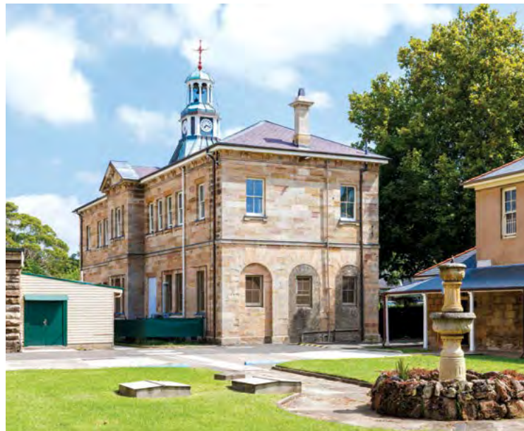
Above: Designed by James Barnet and built in 1874 as the Tarban Creek Asylum Stores and Works building, it is now occupied by Giant Steps Day Care. In 2021-2022 the Program undertook extensive repairs to stabilise sandstone pediments, chimneys and roof framing and reinstate the slate roof. Photograph by Sebastian Mrugalski, 2023.
