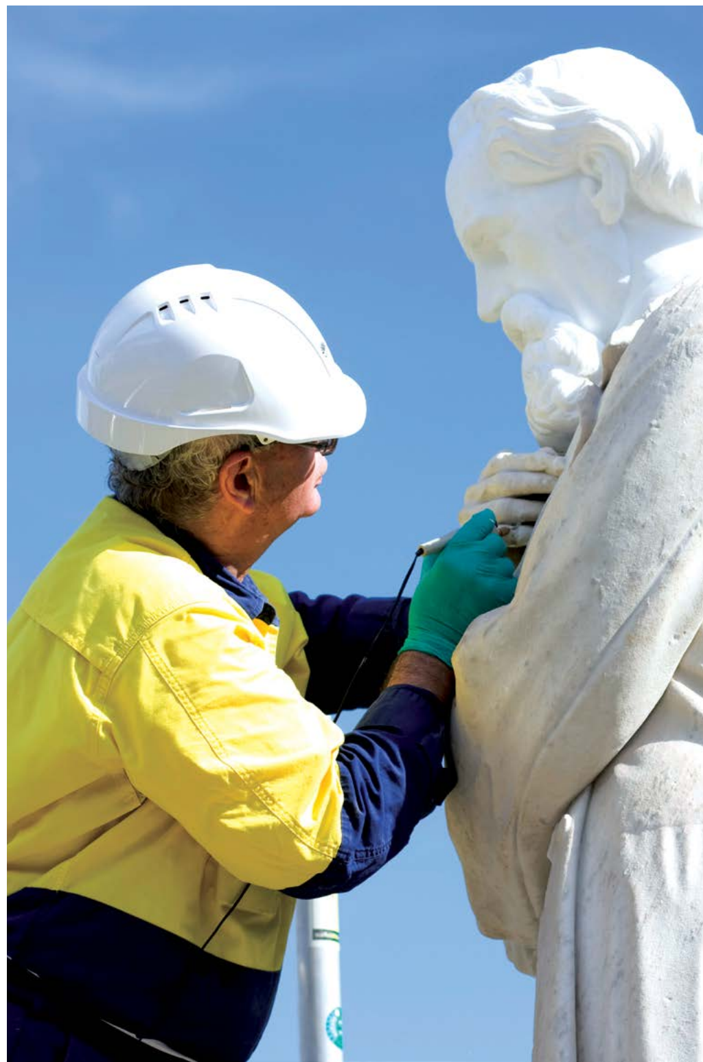
Stonemason Reuben Varfi applies the finishing touches to the statue. A block of carving quality marble was sourced from Carrara, Italy to recarve the head, pen and part of the scroll. The legs were structurally stabilised with pins, the marble was cleaned and the letters were re-leaded using traditional techniques. Photograph by Michael Nicholson, 2011.
