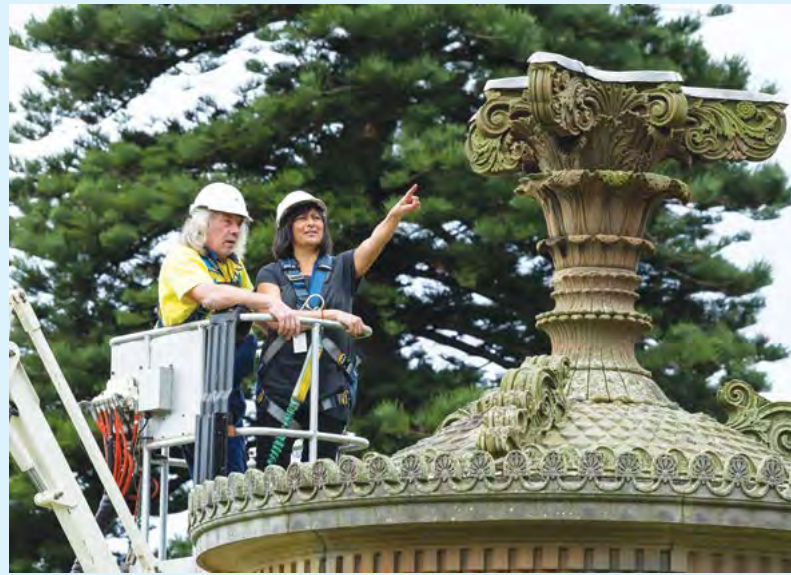
Top left: Carved more than 150 years ago, the Sydney monument's frieze has been adversely affected by the elements and especially salt-laden air. Photograph by Douglas Frost in 2015.
