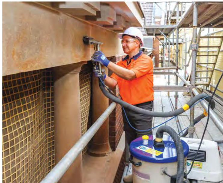
Stone at Fort Street High School, Petersham, is desalinated by Dariusz Piekutowski with a water-captive rinsing system. Photograph by Sebastian Mrugalski, 2023
