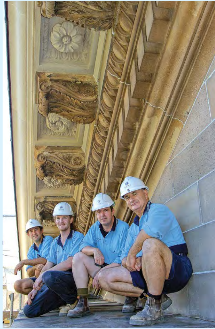
Above: Masons kneel within the College Street pediment, underneath the new rosettes, 2002.
