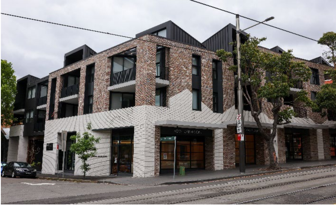
Figure 4. Shop-top housing in Surry Hills
