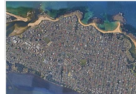
Figure 1. A coastal settlement in NSW displaying many of the common pressures (Nearmap)
