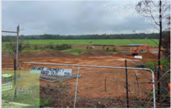
Open trench progress at Wallacia
