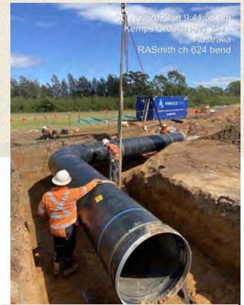
Pipe installation towards eastern end of alignment.
