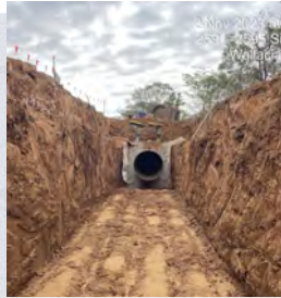
Open trench progress at Wallacia
